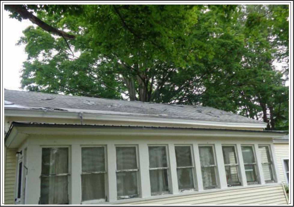
Roof in need of replacement
