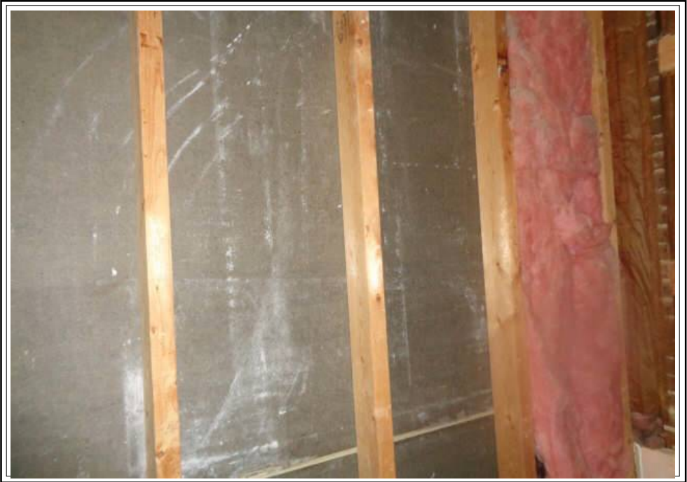
Comment: Missing drywall in bathroom
