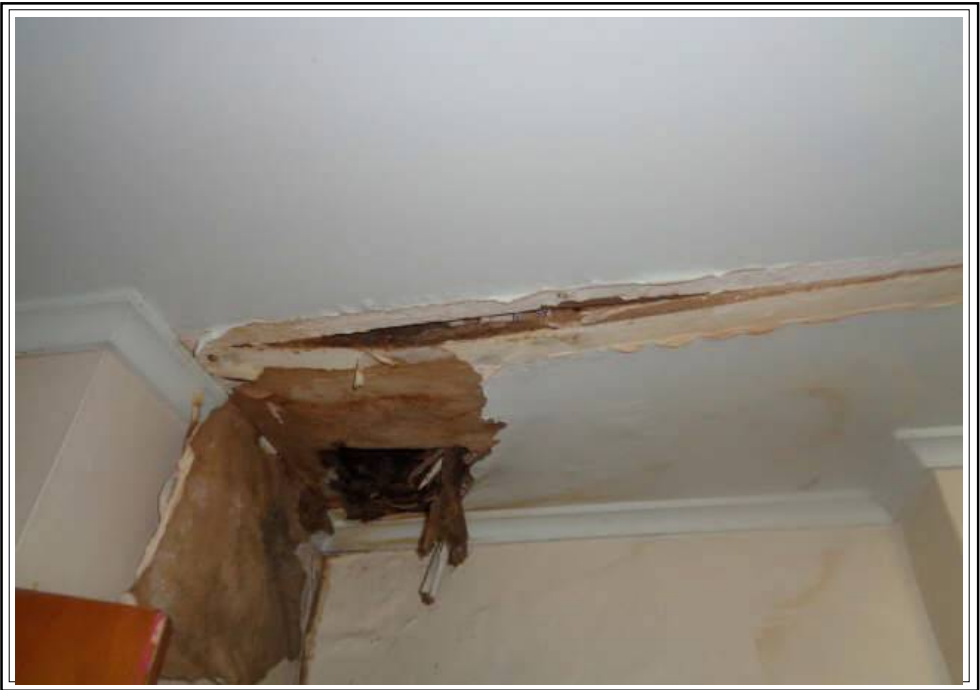
Comment: Damaged drywall in second floor bedroom
