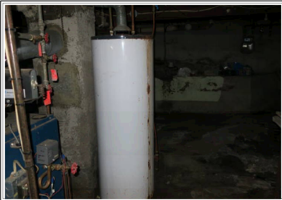
HOT WATER HEATER
