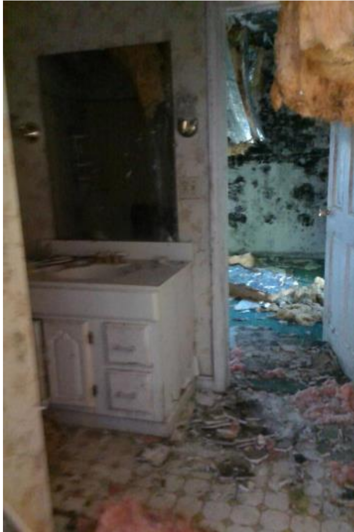
10 WIN_20160912_121231 Date Taken: 9/12/2016 Taken By: Britt Bridges CMR CMI CLR
