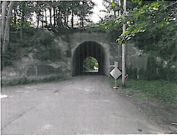
Lake Avenue Viewing Southerly
